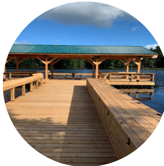
A new fishing dock supports wheelchair users. A shade canopy provides essential sun protection for Campers who are sun-sensitive, especially during treatment.
