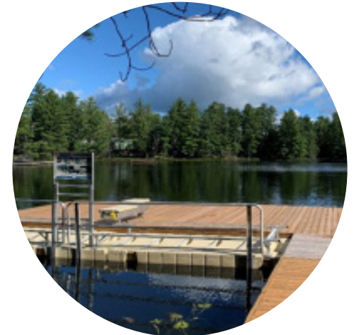
The expanded canoe dock with E-Z launch allows Campers with limited mobility to get into a canoe or kayak safely and independently. Now, a cabin group can launch into the water all at once.
